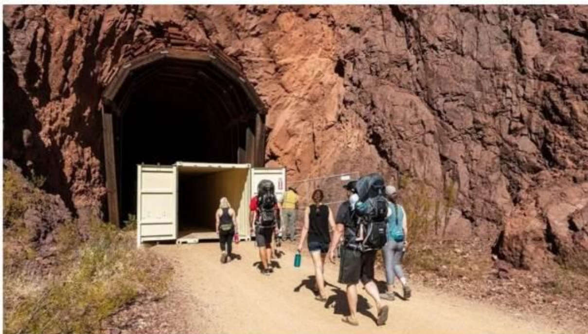
The full Historic Railroad Trail has reopened, though containers have been placed in the second and third tunnels to protect people from falling rocks. (Photo: National Park Service)
