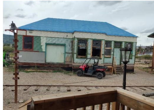
The Dumont Depot sporting a new roof.
